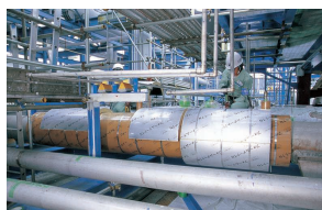
Installation construct of industrial thermal insulation
