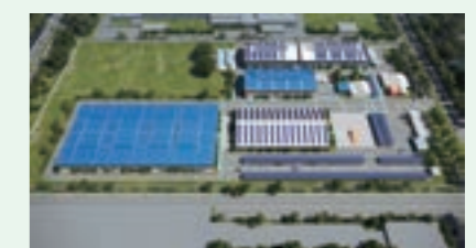
(3) Introduction of solar panels (NT RUBBER-SEALS SDN. BHD. 640kW)
