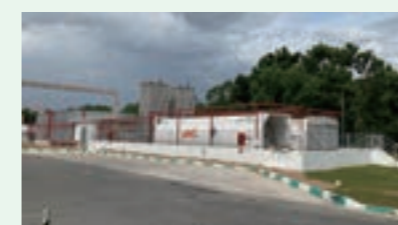
(1) Introduction of LNG storage facilities (NICHIAS FGS SDN. BHD. METAKOTE No.2 line)
