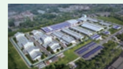
(2) Introduction of solar panels (NICHIAS FGS SDN. BHD. 1,280kW)
