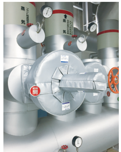
Heat supply plant Steam header valve (Marunouchi Heat Supply, Co., Ltd.)
