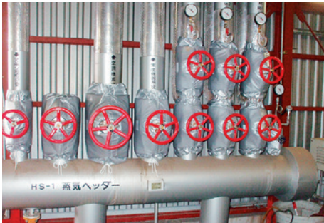
Valves in the boiler chamber and around the steam header
