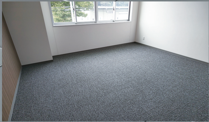
Example of installation (installation of tile carpet)
